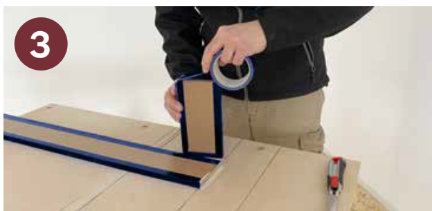
3 MASK THE DECOUPLING STRIPS
