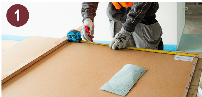
1 MEASURING AND MARKING THE CUTTING LINE
