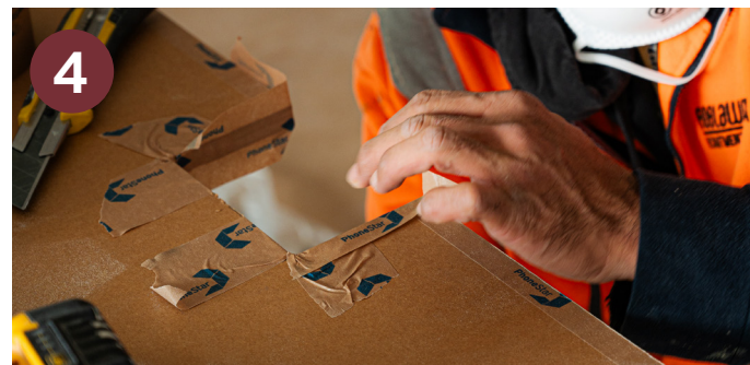
4 FOLD OVER THE CORNERS AND LONGITUDINAL SIDE
