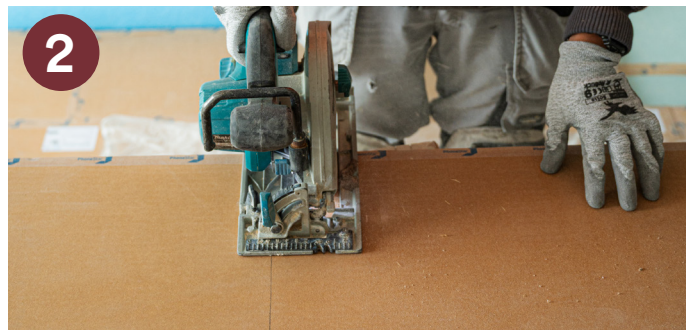
2 CUTTING THE BOARD TO SIZE
