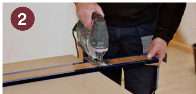
2 CUT THE DECOUPLING STRIP TO SIZE
